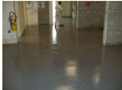
Completed floor finished with epoxy coating
