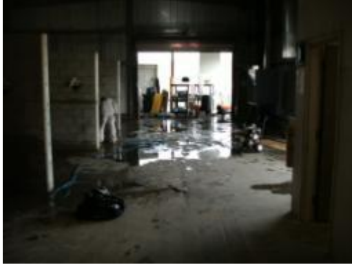
Cleaning and preparing of the concrete surface prior to application of epoxy coating
