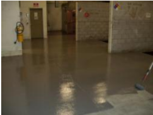
Completed floor finished with epoxy coating
