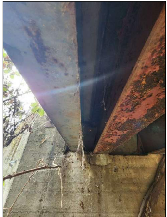
Fig 19: New edge girder added for railing
