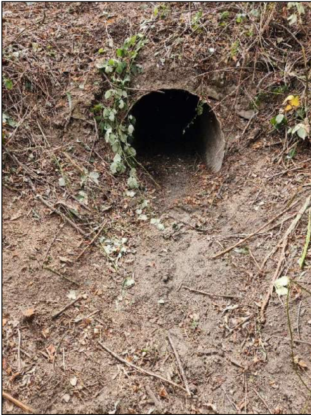
Fig 16: 42" CMP upstream from bridge
