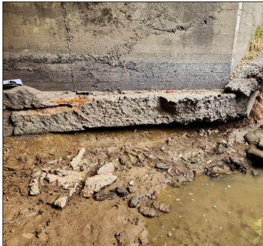
Fig 7: North Abutment Foundation
