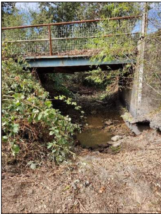
Fig 3: East view of bridge from creek bed
