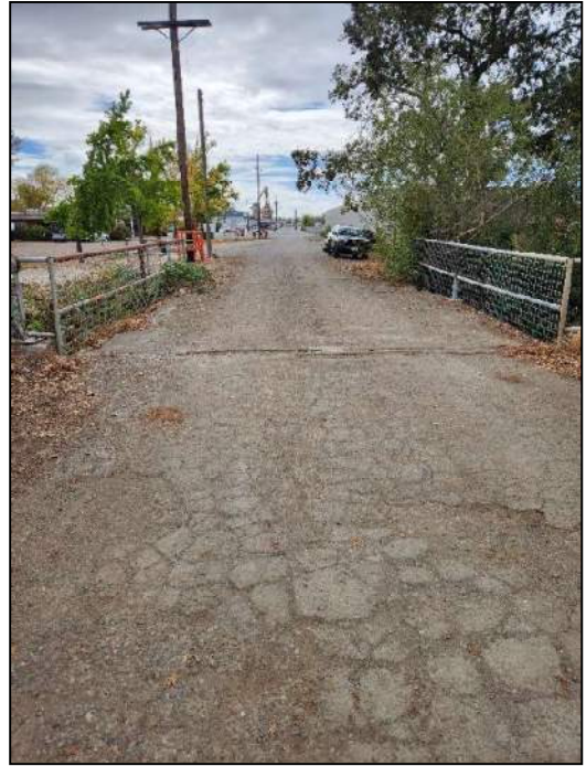
Fig 2: South view of bridge from approach
