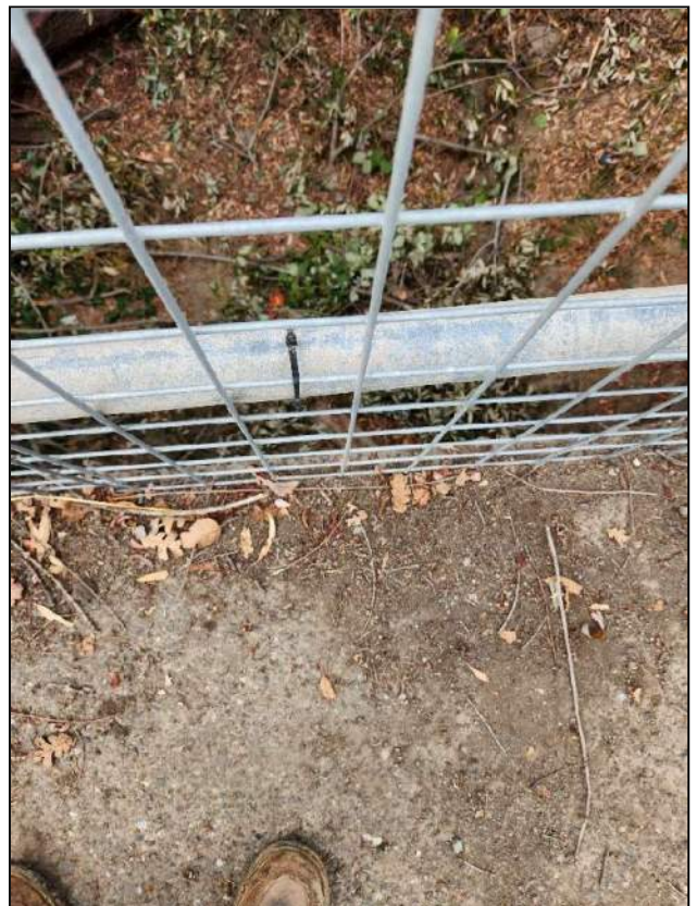
Fig 23: Zipties holding mesh to tube railing
