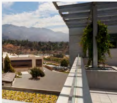
LEED Gold-certified Flight Projects Center facility featuring a living roof and high-efficiency building systems.
