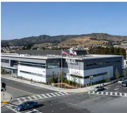
City of South San Francisco Police Operations and 911 Dispatch Center
