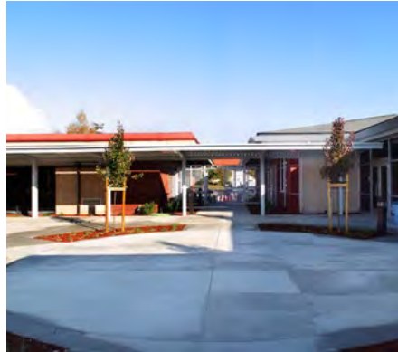
Contra Costa County Public Works Building Expansion
