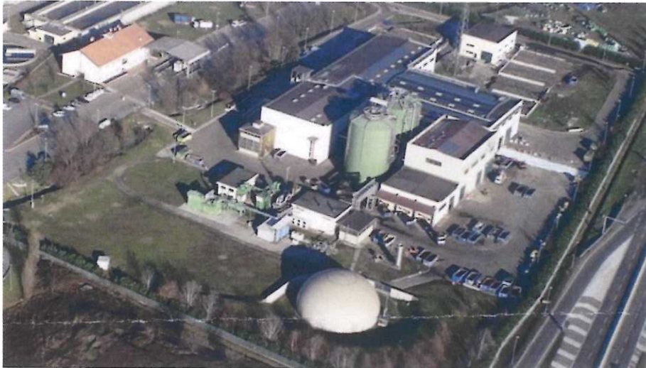
Fig 11: Acea Pinerolese AD composting plant
