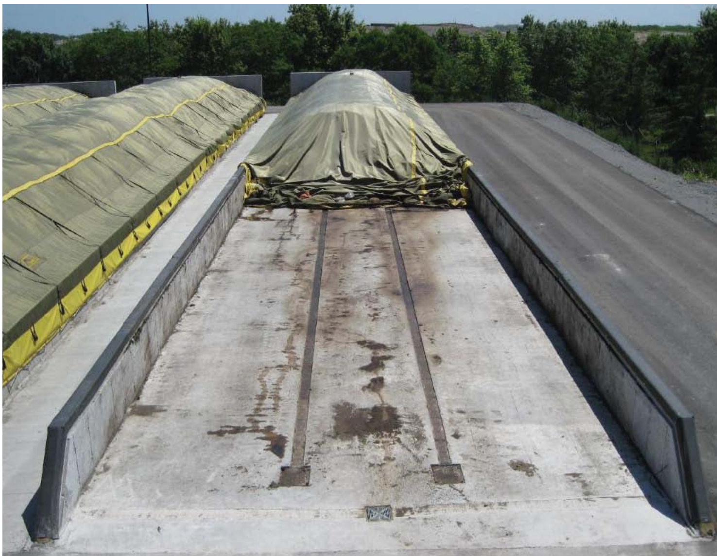
FIGURE 2-4 Typical GORE Bunker Sonoma County Waste Management Agency Compost Facility CEQA Documentation Review
