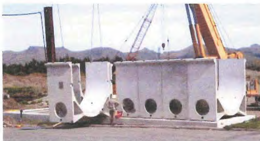
HotRot 3518 concrete modules being installed
