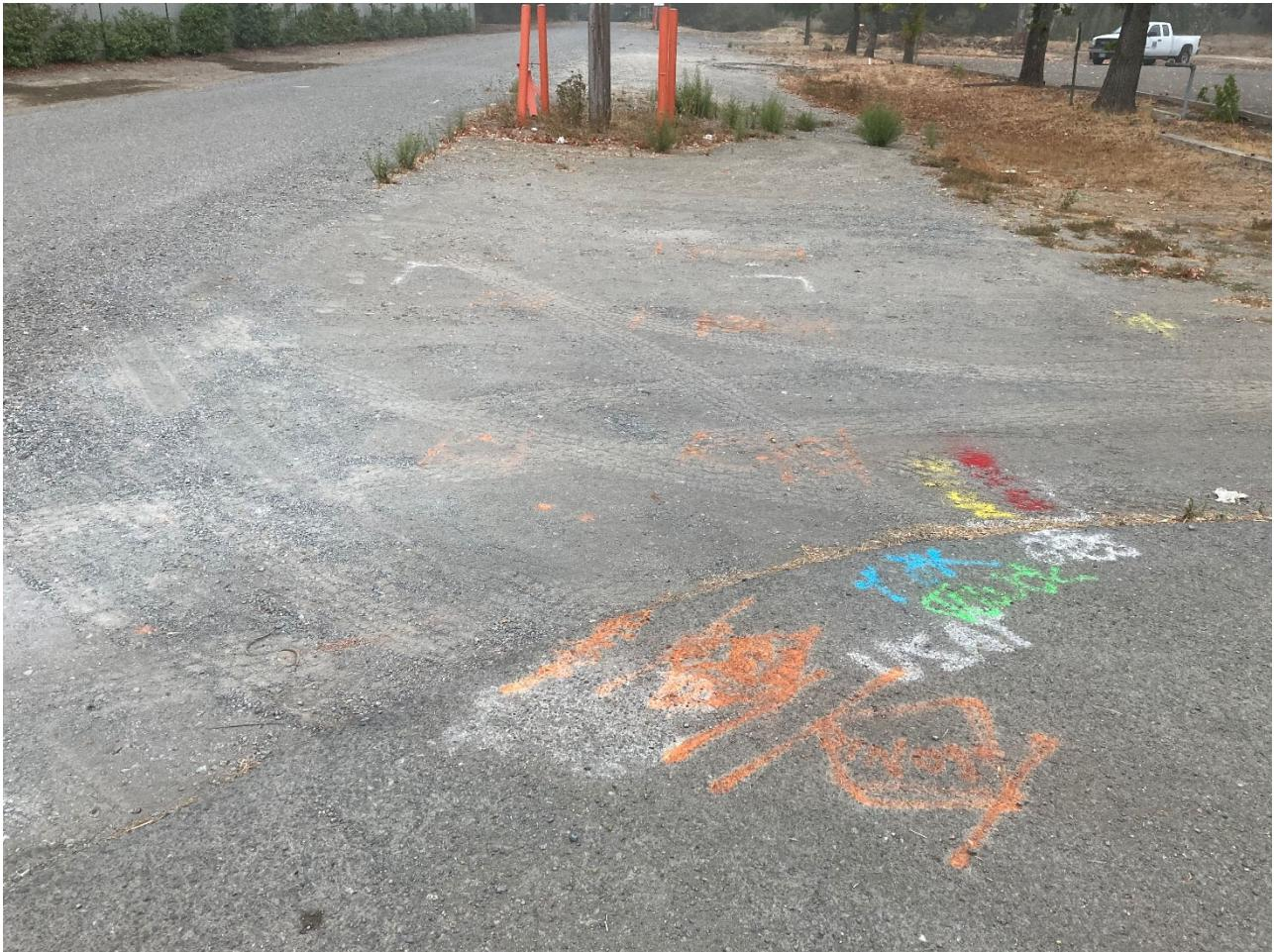
**Comments:** Drilling area at SB-4; hole drilled at edge of roadway to avoid underground utility conflict
