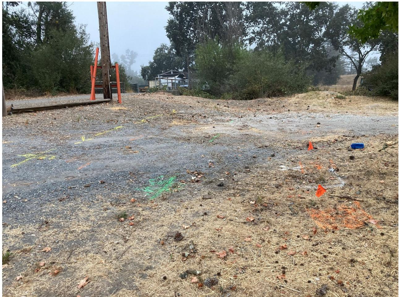
**Comments:** Drilling area at SB-3; hole drilled at left side of image of avoid underground utility conflict.
