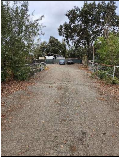
Fig. 1: North view of bridge from approach
