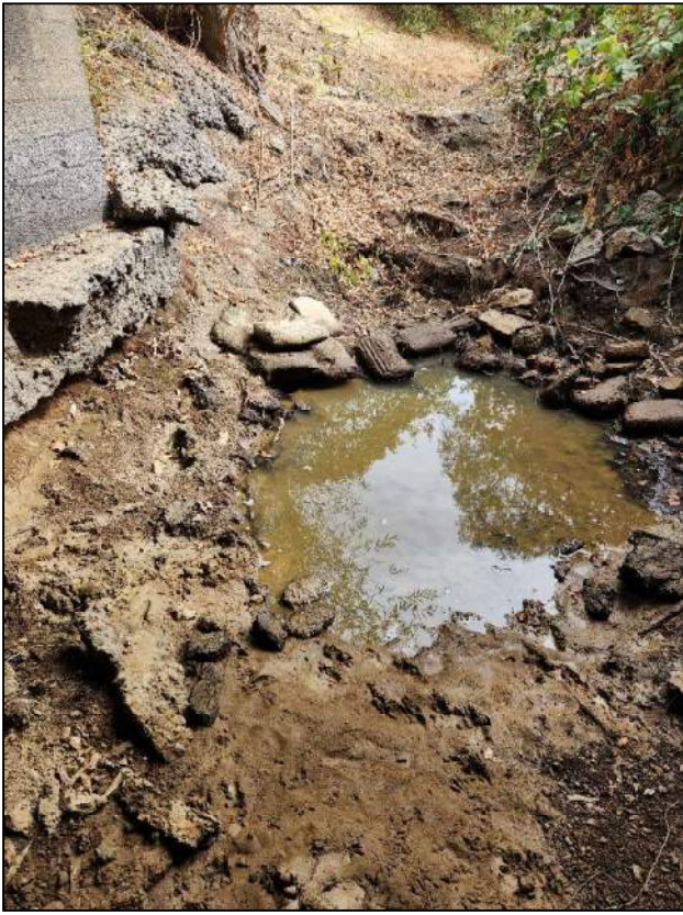
Fig 12: Sacked Concrete in creek bed
