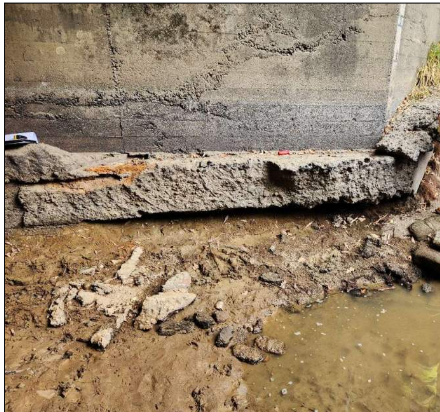
Fig 7: North Abutment Foundation
