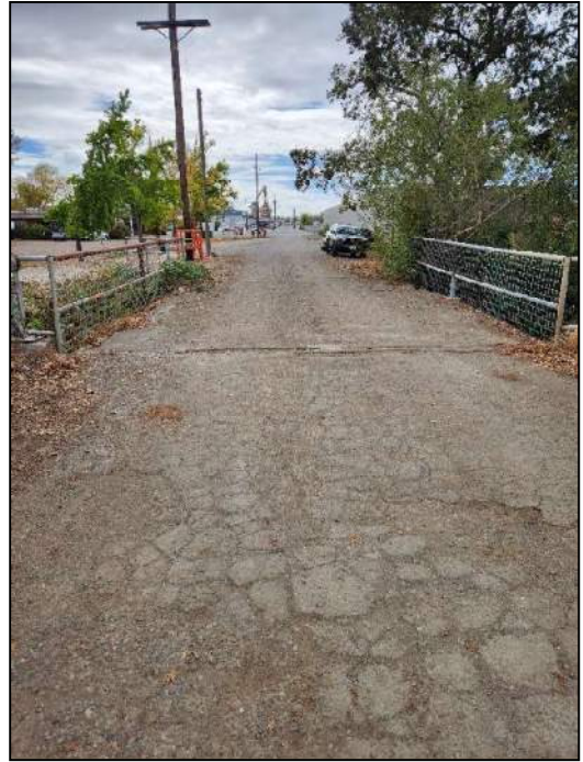
Fig 2: South view of bridge from approach
