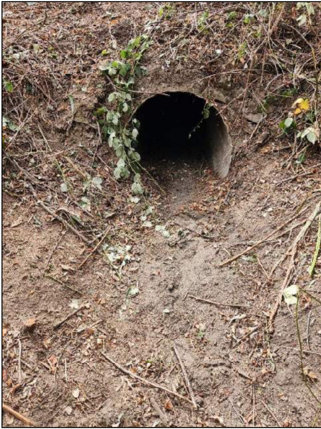
Fig 16: 42" CMP upstream from bridge
