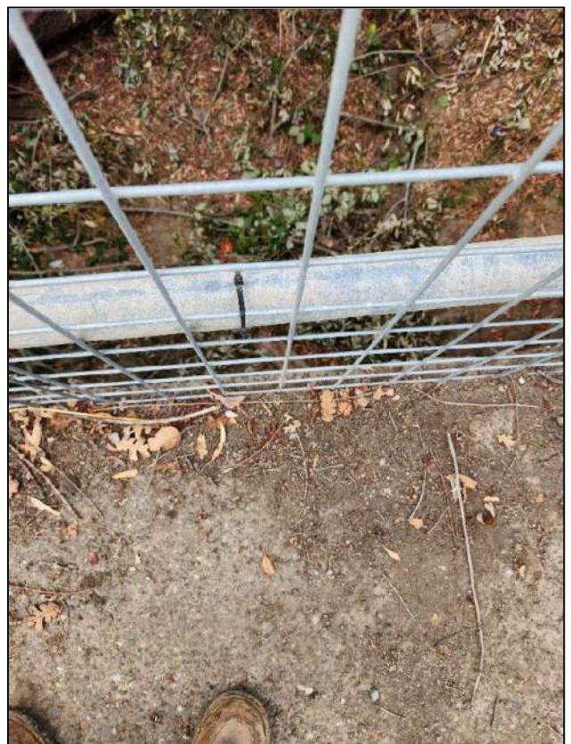
Fig 23: Zipties holding mesh to tube railing
