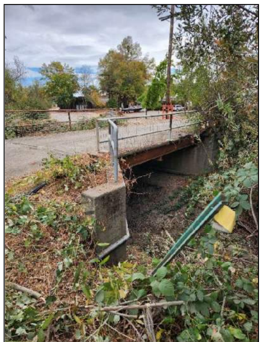
Fig 4: West view of bridge from roadway
