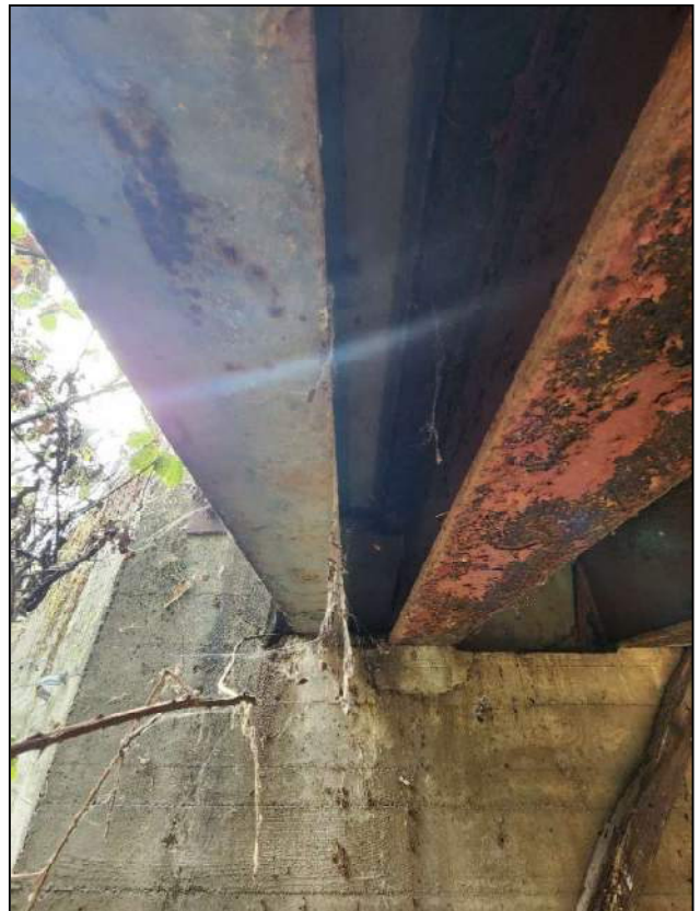
Fig 19: New edge girder added for railing
