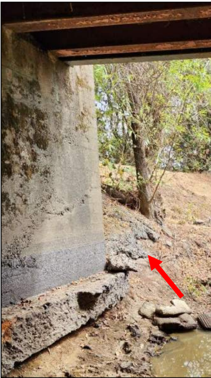
Fig 12: Sacked Concrete in creek bed
